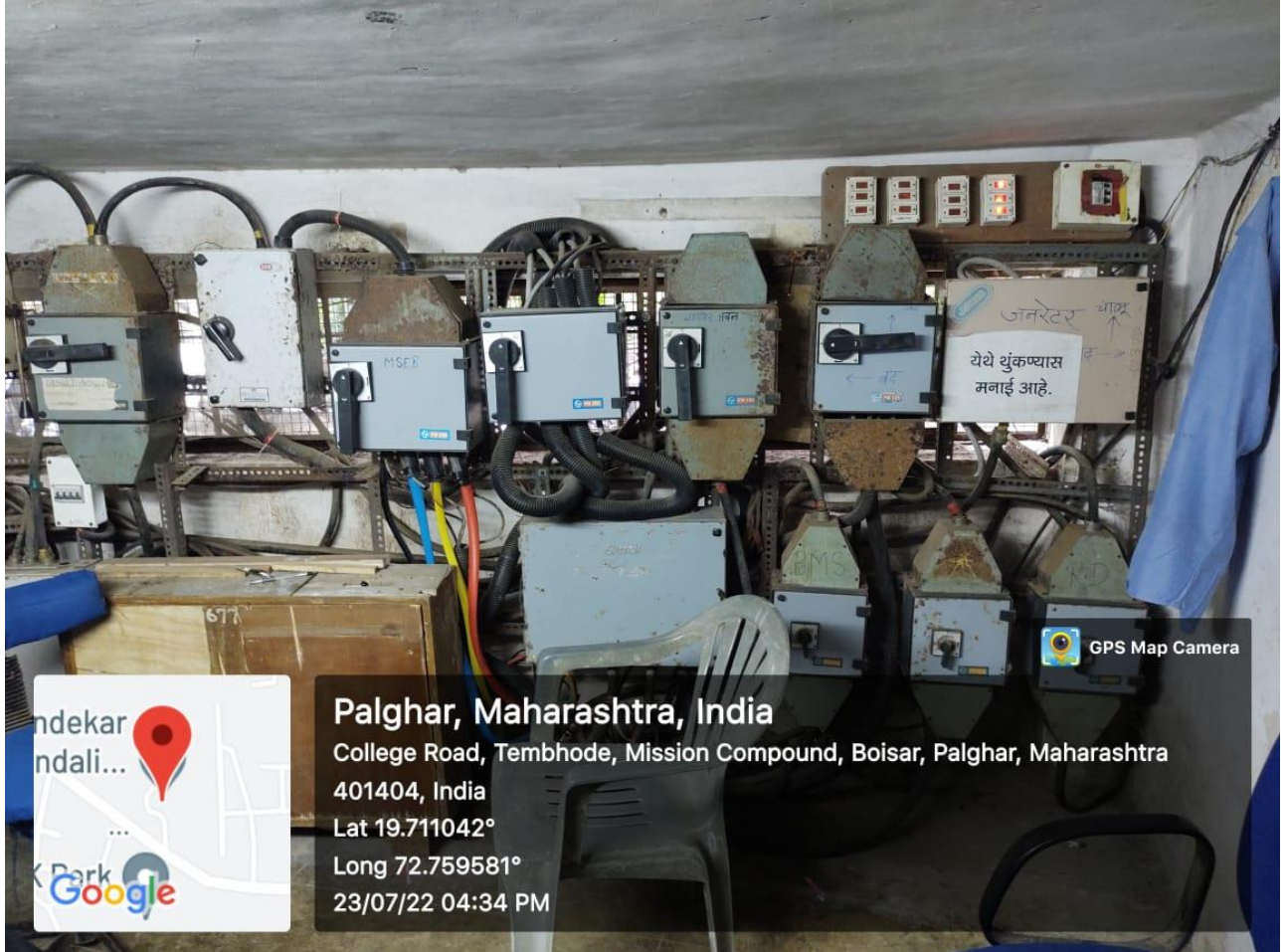
Wheeling to the Grid
